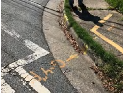
Corner of intersection without ADA compliant curb ramps
