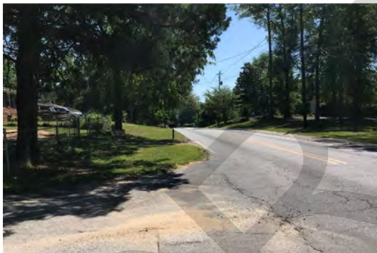
Eastward view from Englewood Drive blocked by crest
