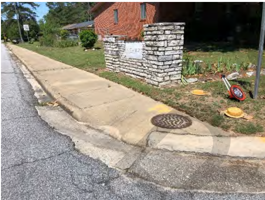
Curb ramp angled toward Steam Mill Road at Bowen Boulevard
