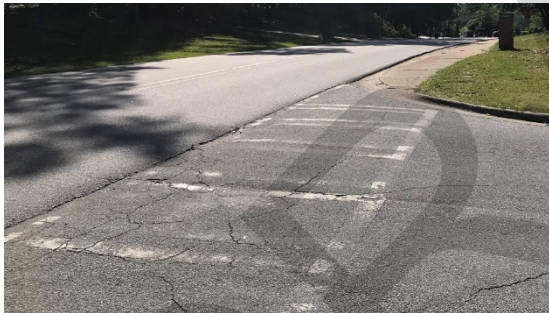
Faded crosswalk at Chandler Drive intersection
