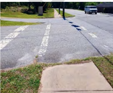
Curb ramps across Shirley Winston Park Driveway without ADA warning surfaces
