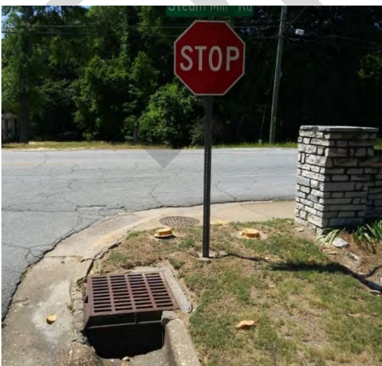
Drainage structure which reportedly floods during storms
