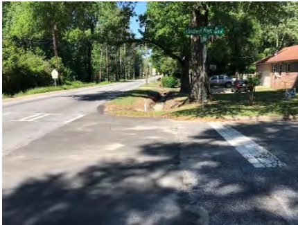
Northwest corner of intersection with no receiving sidewalks or curb ramps
