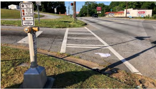
Crosswalk without connecting ADA ramps or sidewalks
