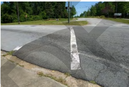
Crossing of western leg without receiving curb ramp or sidewalk
